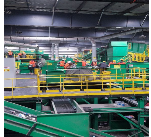
Escondido Resource Recovery
